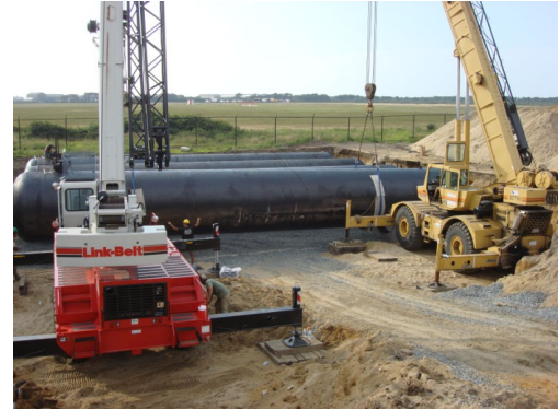
INSTALLATION OF THE (4) 30,000 GALLON TANKS...ALL UNDERGROUND
